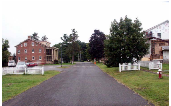
Existing gate and extant buildings
