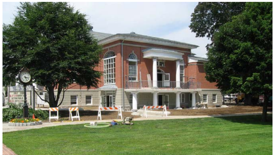
Photo during construction.
