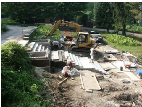
During restoration, June 27, 2003
