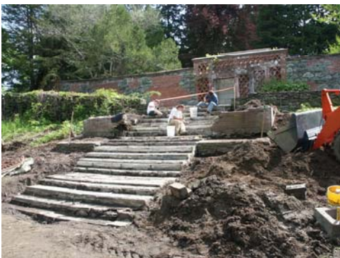
During restoration, May 30, 2003
