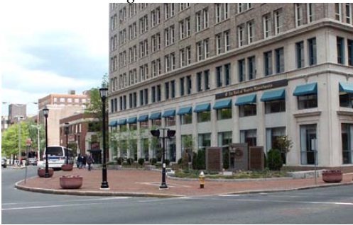
Two years after construction
